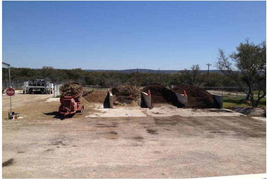
KMUD Compost Facility
