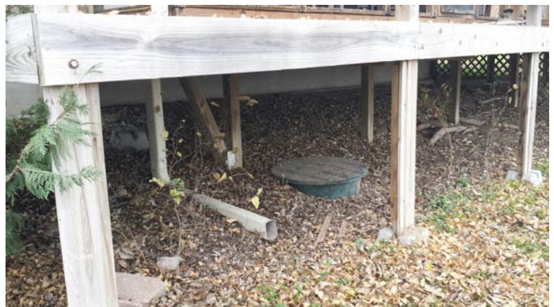
Do NOT place concrete, or any other similar obstructions around the tank. Do not enclose or brick in the panel. The conduit from the panel to the tank (above) is obstructed and inaccessible for replacing. Do NOT place a deck or other obstruction over the tank (see below).
